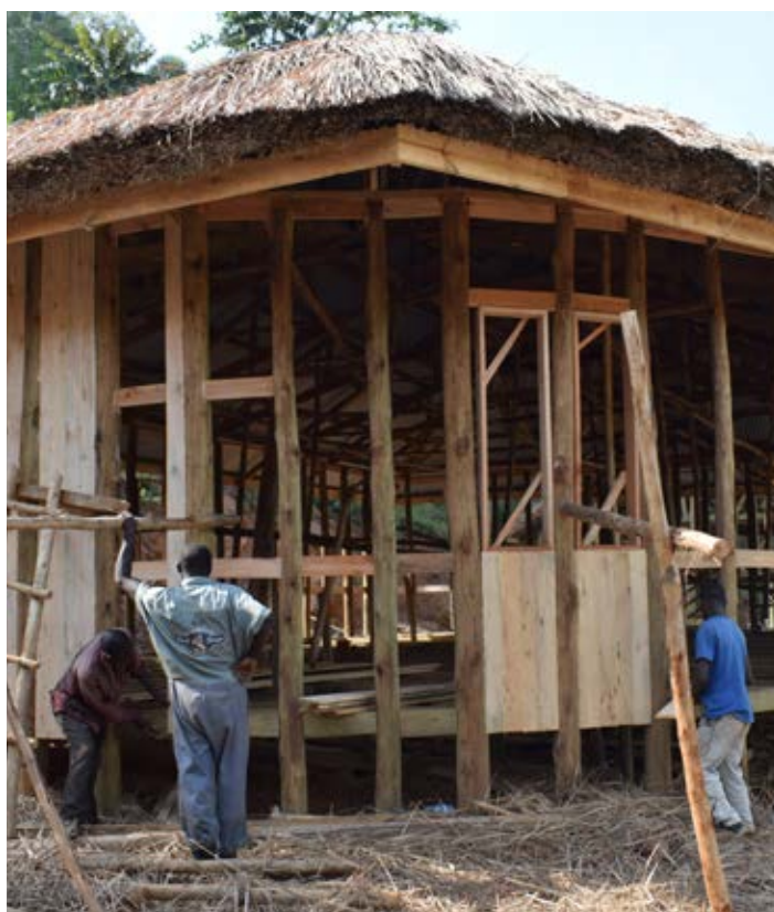
Mbarara University Gorilla trekking camps under construction
